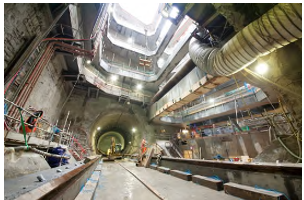
Temporary cradle on which running tunnel TBM would be jacked through Stepney Green cavern on the Crossrail project
